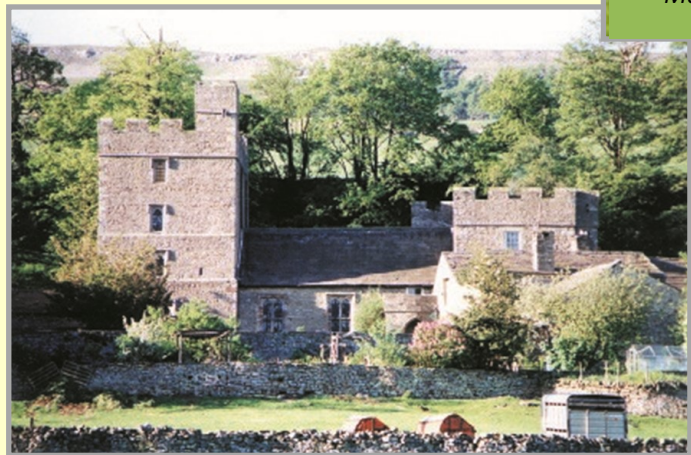
Nappa Hall, Wensleydale, ancestral home of the Metcalfes, originally built c. 1459
